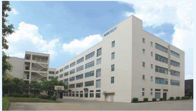
R&D Center in Guangzhou
